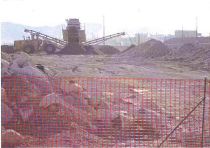
CAMU: Power screening of impacted soils.
