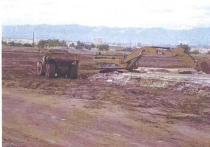
Eastside: SW-3 Loading out wet material.
