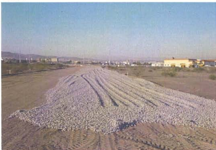
Eastside: Additional trackout rock being installed..
