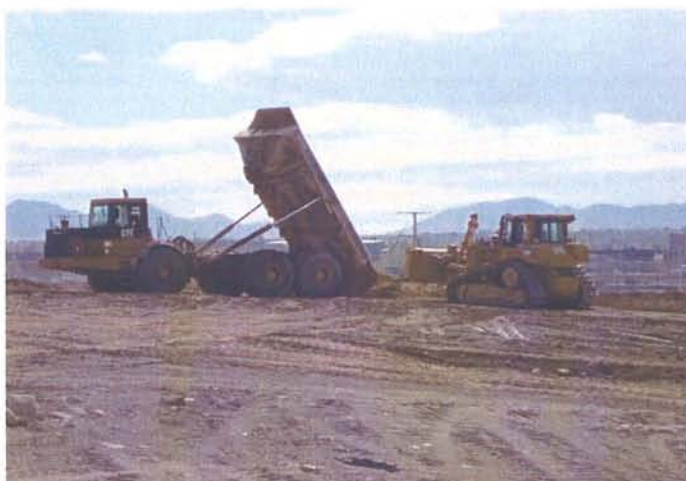
CAMU: 40 ton dump truck. Dumping soils on 200,000 cy stockpile.
