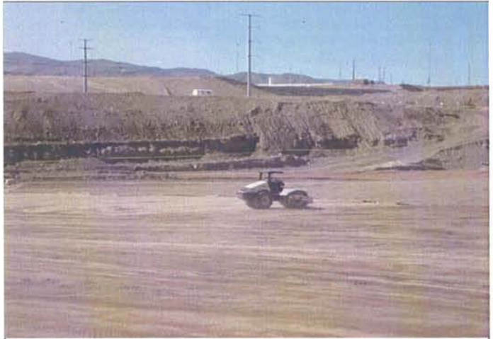
CAMU: Phase 1 compacting waste with roller.
