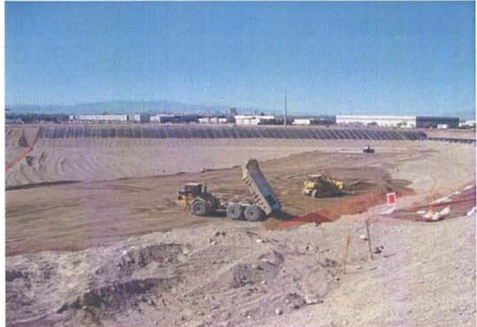
CAMU: Phase 1, Western Ditch soils placement.
