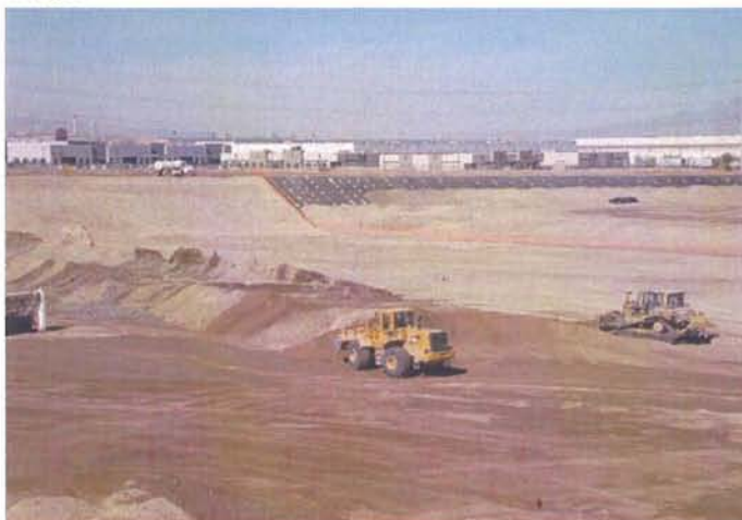
CAMU: Phase 2. Western ditch grading
