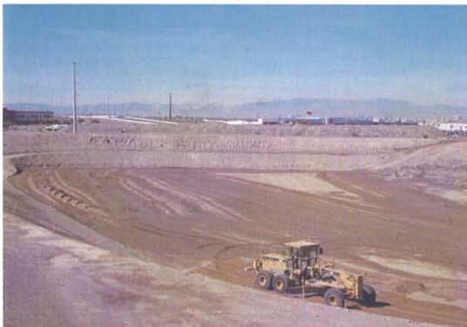
CAMU: Phase 2. Western ditch grading the floor.
