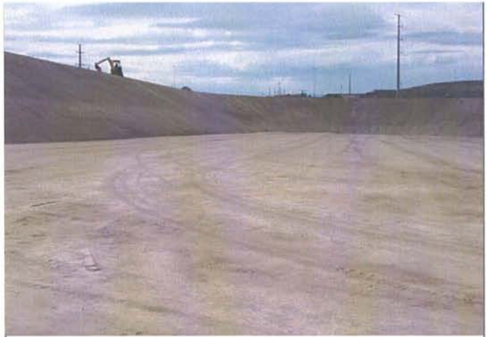
CAMU: Phase II, slopes looking southwest. Backhoe digging anchor trench.
