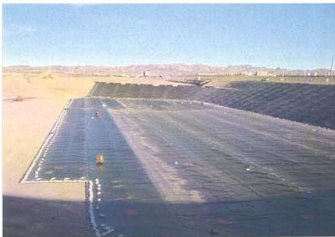
CAMU: Phase II liner being installed on floor.
