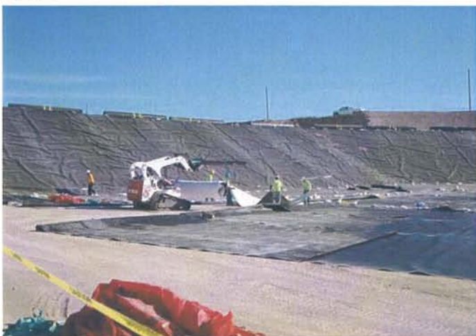
CAMU: Phase II, GCL Liner being installed.
