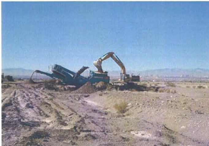
Eastside: Powerscreening moisture conditioned soils at PUB-3
