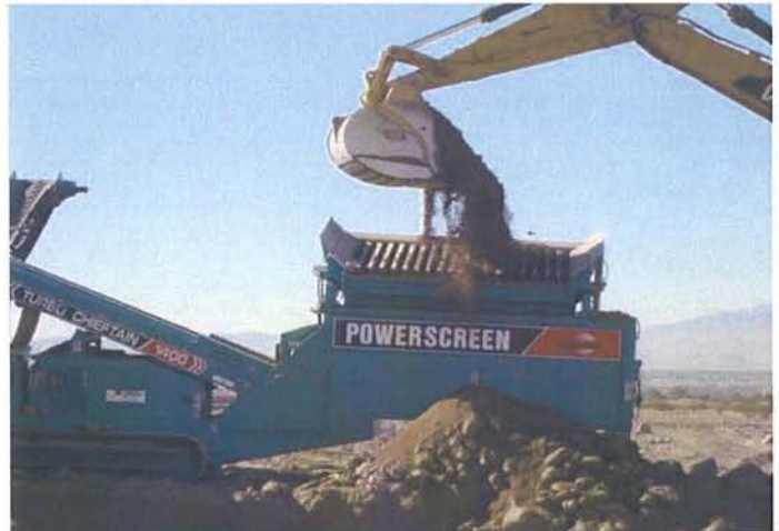
Eastside: Powerscreening moisture conditioned soils at PUB-3.
