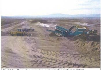
Eastside: Screening operation and sprinkler system moisture conditioning. PUB-4 and PUC-4.
