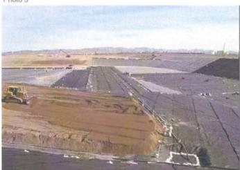
CAMU: Phase II operation layer grading off top for LCRS pipe and rock installation.
