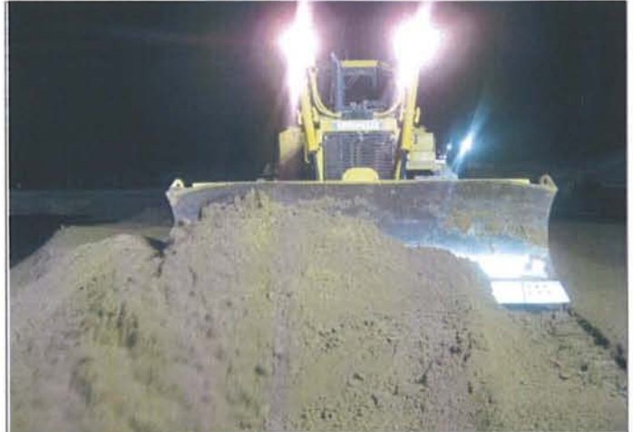
CAMU: Phase II , Operations layer material being placed with D6 dozer. With oversight.
