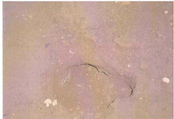
CAMU: BMI North Landfill, small sink hole discovered and properly compacted..
