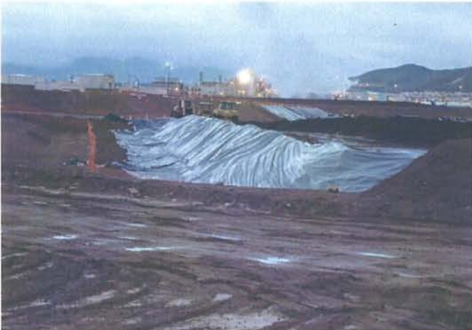
CAMU: Phase I, Iterim cover with visqueen plastic. North slope.
