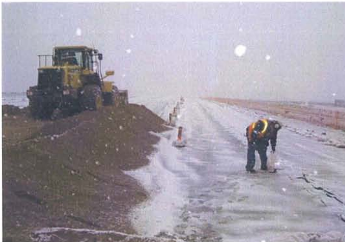
CAMU: BMI North Landfill. Work stopped placing operation layer due to temperature.
