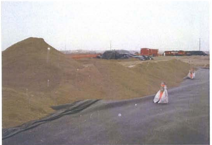
CAMU: BMI North Landfill, beginning of operations layer placement.
