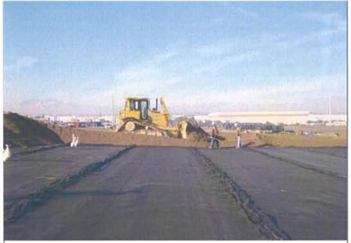
CAMU: BMI North Landfill, placement of 1 inch minus.
