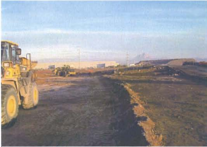
CAMU: Phase IIIB, 6 inch scrape.
