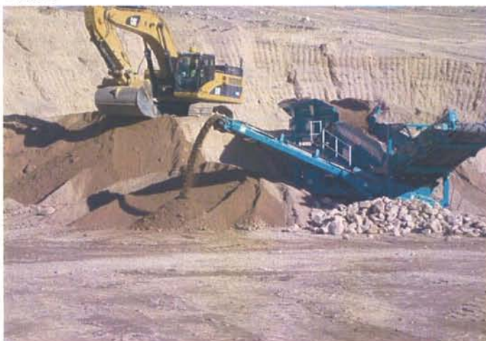
CAMU: Screening operation at 200,000 cy stockpile.
