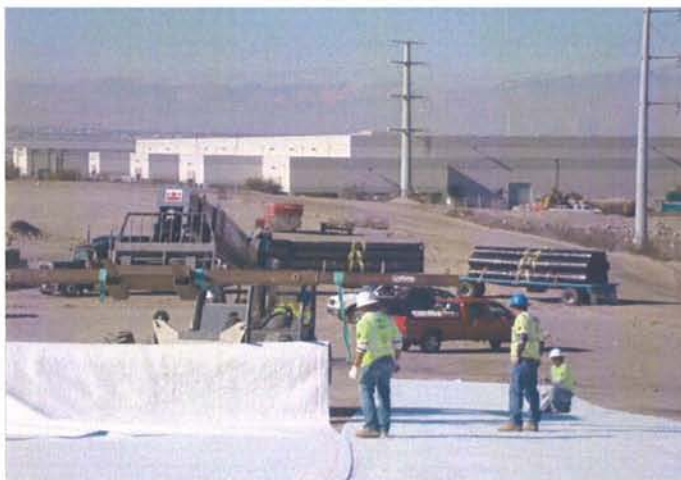
CAMU: North BMI Landfill GCL Liner installation.
