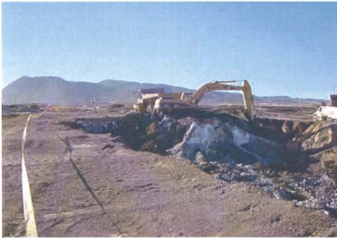
CAMU: NW Basin/Phase IIIB excavation, first 8 foot cut.
