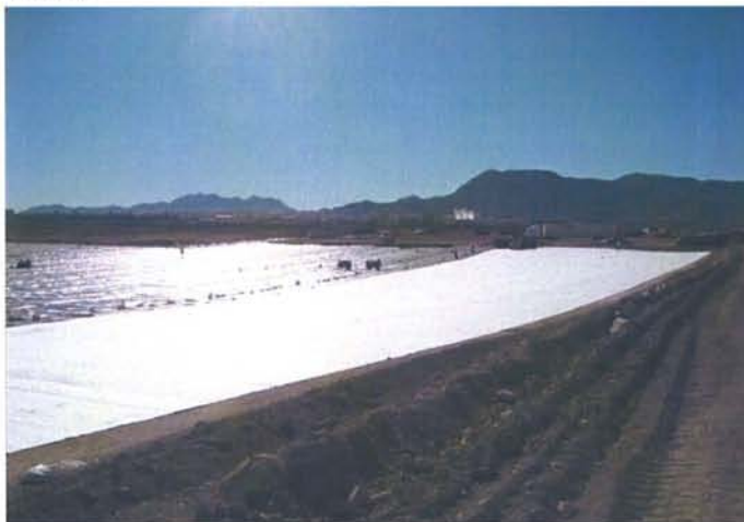
CAMU: North BMI Landfill liner installation.
