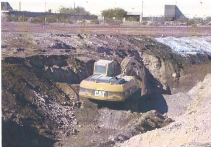
CAMU: NW/Phase IIIB trench excavation.
