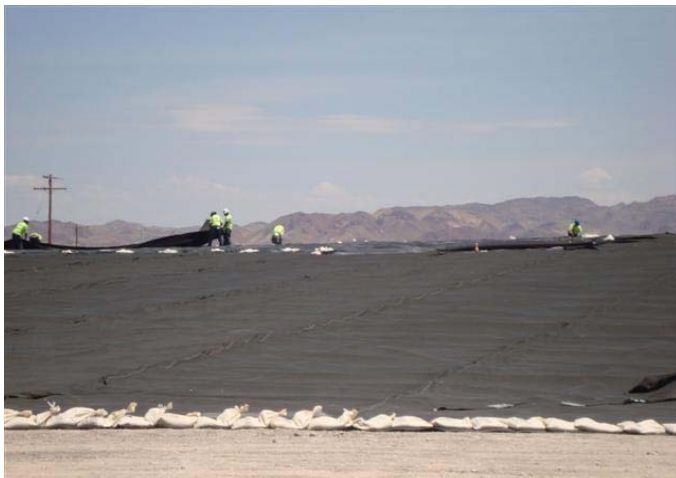
CAMU: ESI installing geocomposite on the South BMI Landfill.
