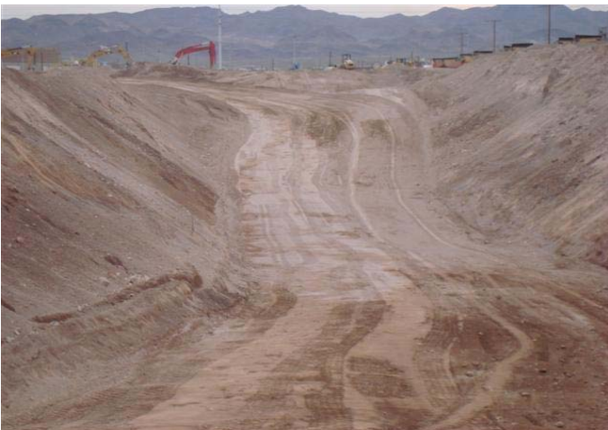
CAMU: SW-1, Slit trench, backfilling.
