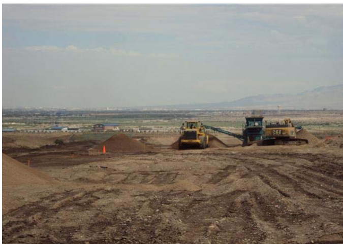
Eastside: Powerscreening beta ditch soils.
