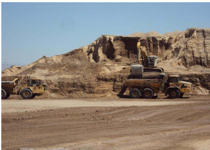
CAMU: Loadout from the 200,000cy stockpile.
