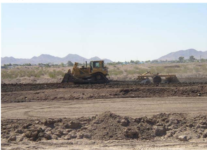
East side: Discing material in PUA-10
