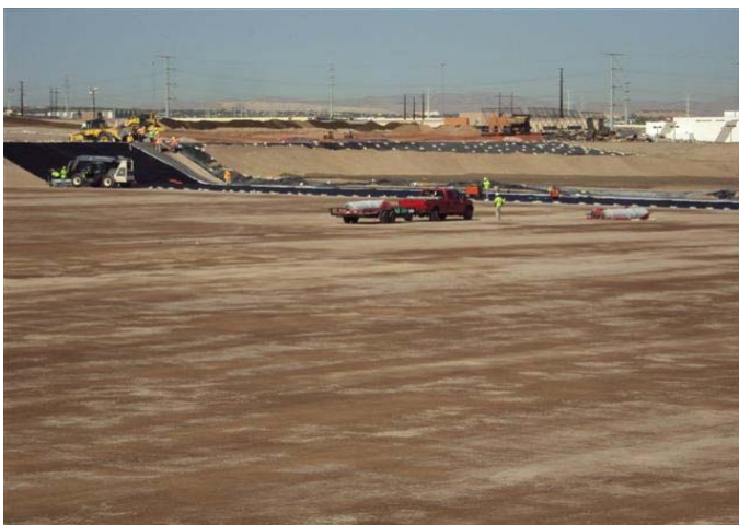
CAMU: Phase 4 GCL and geomembrane installation
