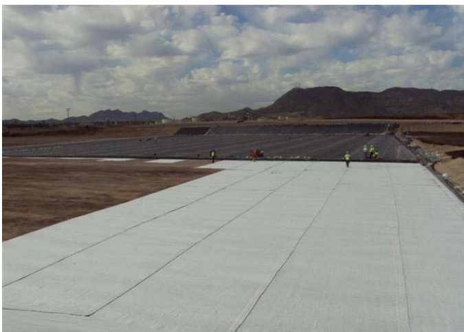
CAMU: Phase 4 GCL and geomembrane.
