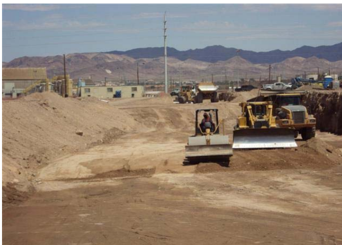
CAMU: Backfill of SE-1.
