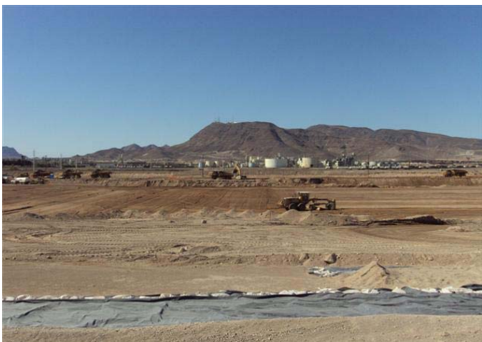
CAMU: Grading on the floor of Phase V.
