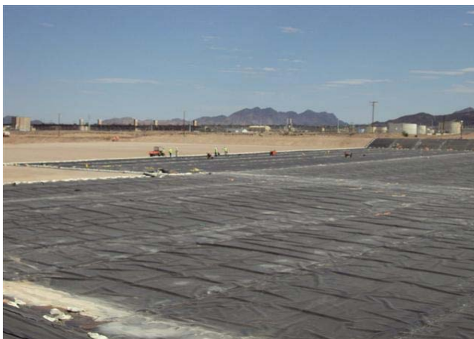
CAMU: Phase IV Liner installation.
