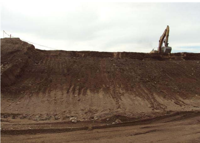
CAMU: Phase V, North Slope Additional three foot removed of brick and debris.
