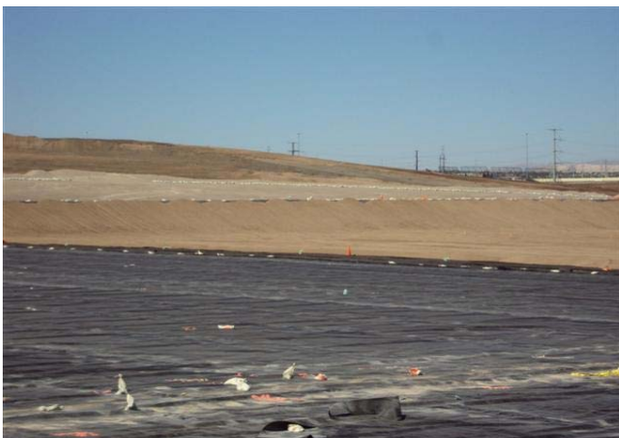
CAMU: Phase IV, liner installation, and operations layer.
