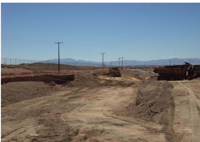
CAMU: SE-2, slit trench, backfill and haul road realignment.
