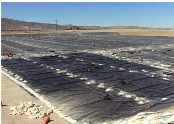
CAMU: Phase IV, liner installation.
