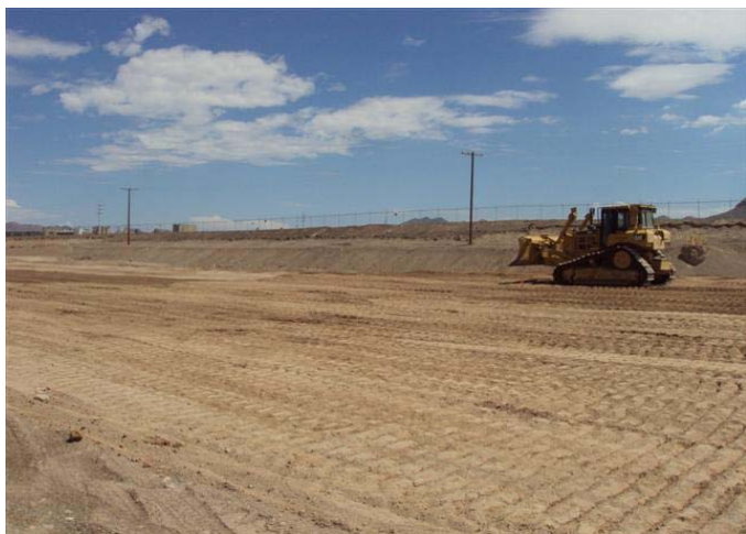
CAMU: Phase V, SE-1, slit trench backfill.
