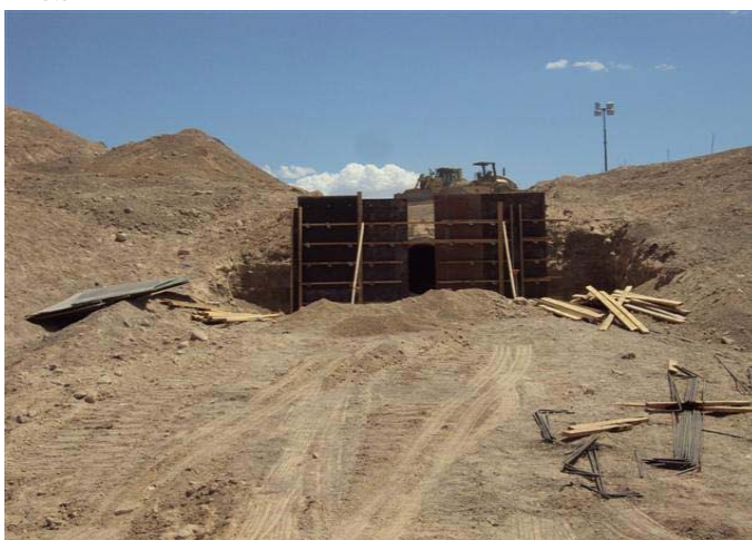
CAMU: Forming headwall, NW detention basin.
