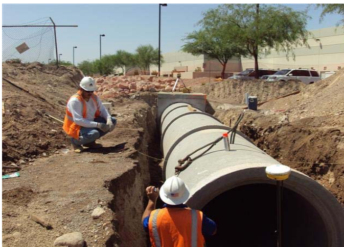
CAMU: 60" RCP installation. MH 8 to Headwall 3.
