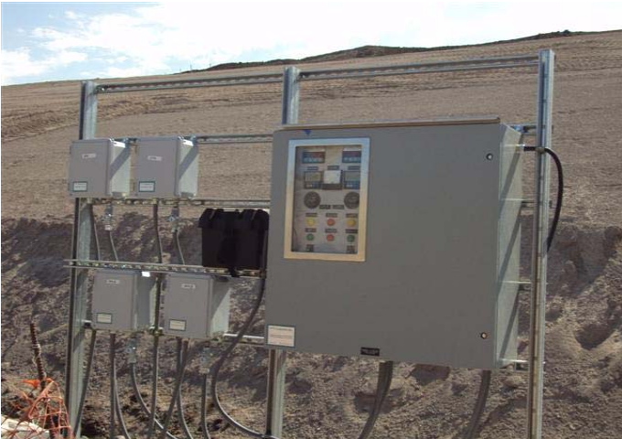
CAMU: Control panel for leachate sump and vadose zone.
