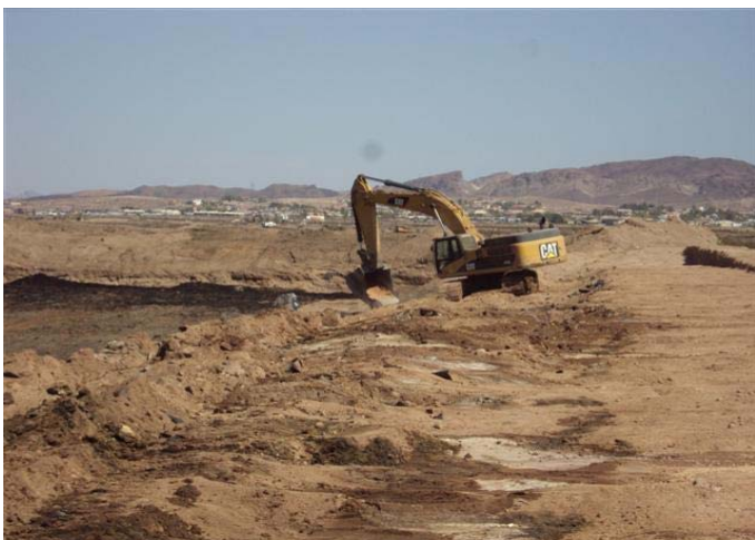
Eastside: Dry ponds excavation.
